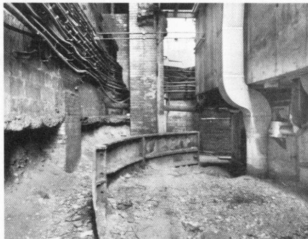
Top of the filled emergency stairs shaft. Photo by Nick Catford
